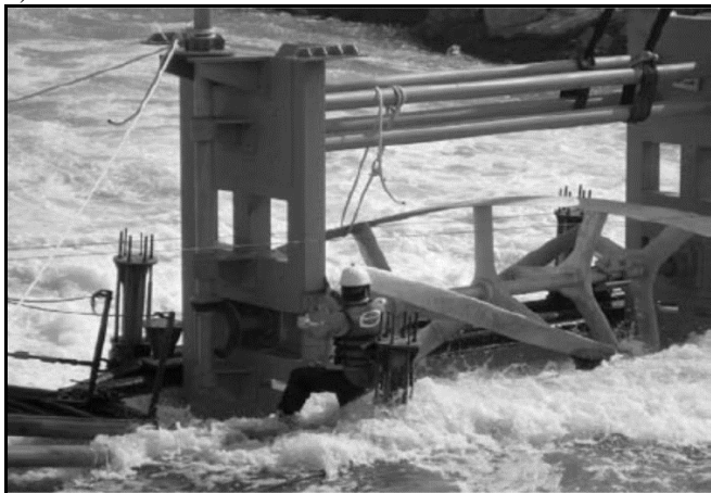
Fig. 1. GHT being installed in South Korea.
