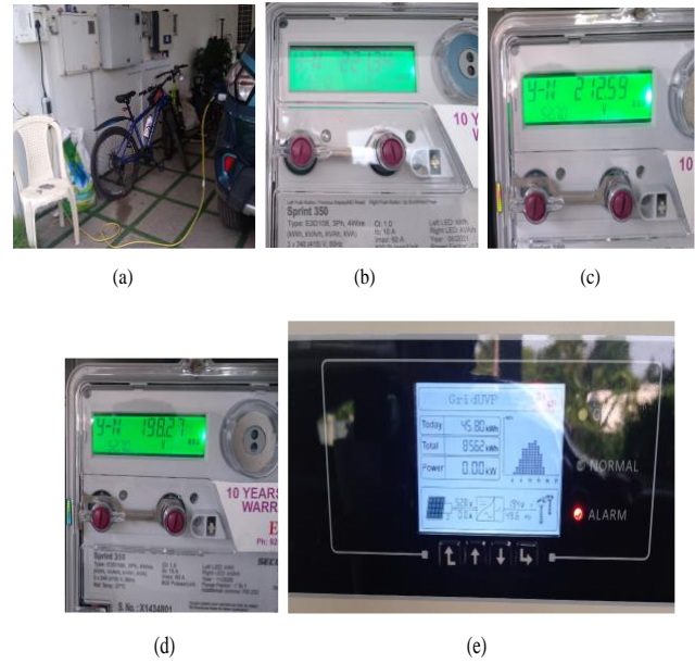
Fig. 7. (a) Charging process of the TATA Nexon EV car; (b) KSEB line voltage with PV integration; (c) Line voltage when EV connected to the same phase for charging; (c) Voltage drop during charging; (d) Inverter display with alarm indication.
