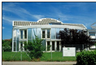
Fig. 5. Self-Sufficient Solar House (SSSH) in Freiburg, Germany (Bond, 2005).
