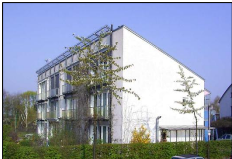
Fig. 2. Passive House in Darmstadt Kranichstein (Feist, 2006)
