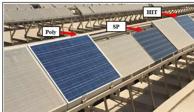
Fig.10. Installed PV Modules covered by dust [KISR].
