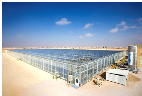
Figure 6. Photo of the solar EOR facility installed in the Mckittrick oil field, USA (image source: https://en.wikipedia.org/wiki/GlassPoint_Solar#/media/File:GlassPoint_EOR_Kern_County_CA/jp ).
