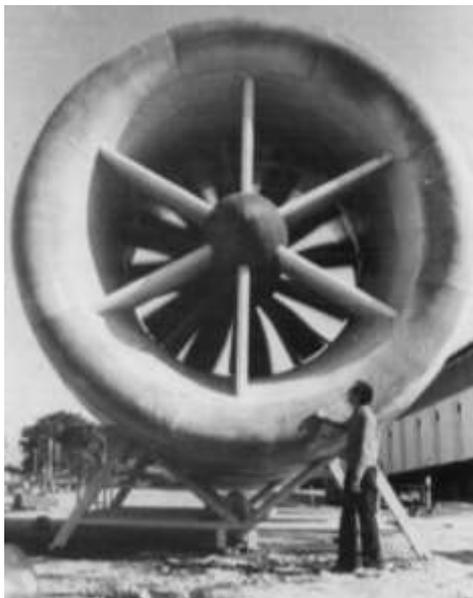
**Fig. 5.** The Pilot Plant for Igra’s Turbine. ‘ $q$ ’ refers to volumetric air flow rate ( $m^3/s$ ) [19].
